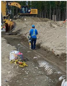
To suit virtually any application, Hi-Flo® Round Pipe and Pipe Arch come in many different diameters and lengths of 6 m or longer. Thicknesses range from 1.6 mm to 2.8 mm. Hi-Flo® is about 1/12th the weight of concrete pipe.
