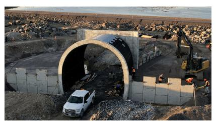
To resist the ice-force on the downstream side facing Hudson Bay, that headwall was backed by a thick, cast-in-place concrete wall which was reinforced with flat sheets of Bolt-A-Plate. And, to avoid corrosion from salt water, plastic geogrid was used for the MSE soil reinforcement on both headwalls.
